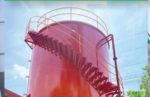
ABOVEGROUND WATER TANK
